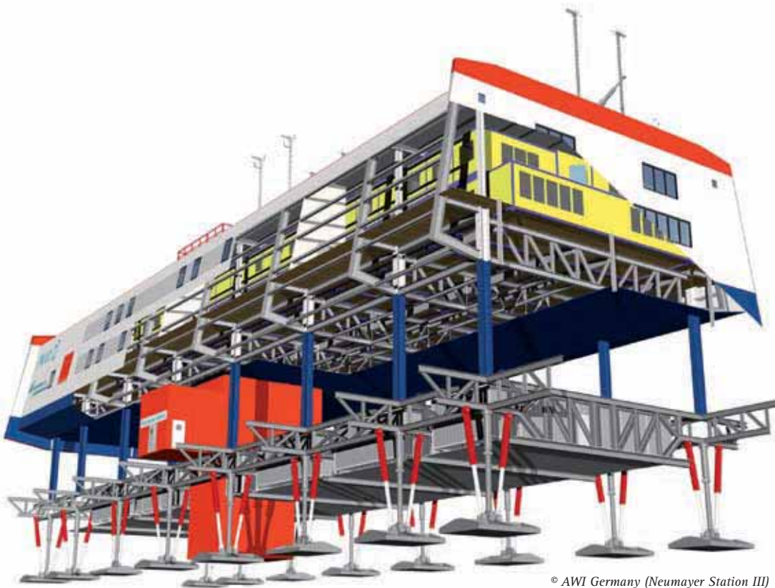
© AWI Germany (Neumayer Station III)
